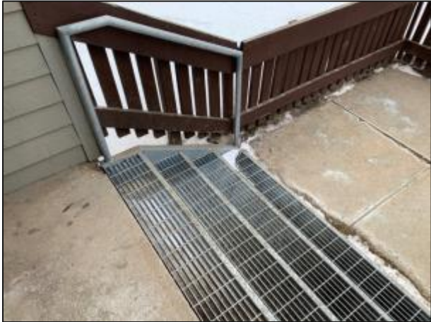
Upgraded & Repaired Stairs
