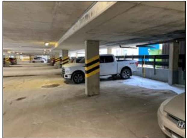
Lower Level Parking
