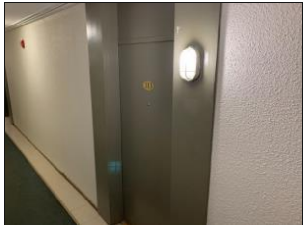
Typical Unit Entrance
